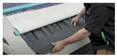
**STEP 1**To install the felt support tray, position on top of the fascia board and fix into place using clout nails.
