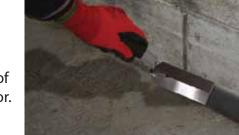
Alternatively apply KA Fillet Seal to a height of 25mm and horizontally 25mm across the floor.
