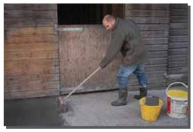
Tanking can be poured, brushed or trowelled in one application to a depth of 3-5mm.
