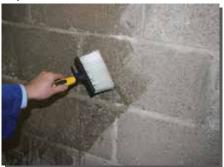
KA Tanking must be applied to a porous, wet, cementitious substrate including brick, block, concrete and stone.
