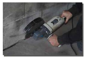
Where floor meets wall make a saw cut approx 15mm deep at 45°. Make sure the tanking flows into the cut when applying the tanking.
